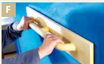
F Flat grinding of large areas
