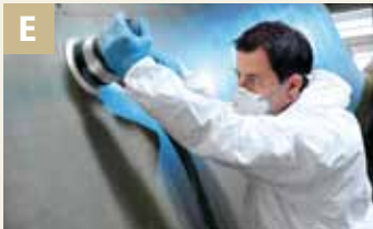
E Keying/flat grinding of rough surfaces
