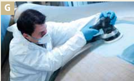
Flat grinding/fine sanding of epoxy filler
